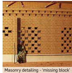
Masonry detailing - 'missing block'
