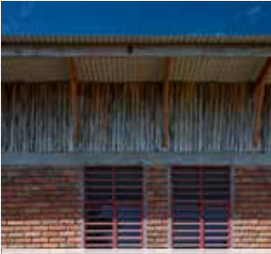
Profiled metal sheet & shuttered
